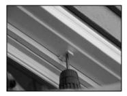
**2** – Grasp side rails and insert the bottom internal lock end caps. Next, insert both side rails onto protruding edge of housing end caps. Align rails plum into final position on window and fasten to window frame using screws.
